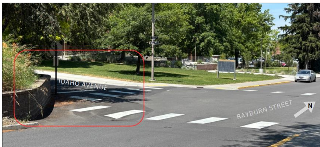
Existing conditions show the north/south crosswalk is set back farther into Idaho Avenue in conjunction with a short retaining wall and topography
