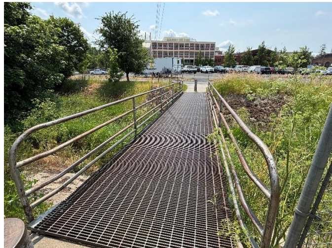
The existing Pedestrian Bridge at the southern extent of Home Street. The bridge deck is too narrow, sits too low within the flood plain, and the handrails/guardrails are not code compliant and are unsafe.
