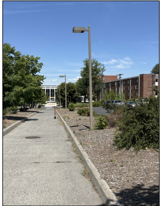
Existing conditions of the walk path illustrating the cracking concrete, old direct-bury lighting, along with missing/remaining vegetation.
