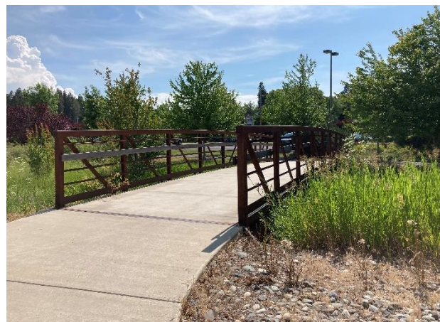
Existing Prefabricated Pedestrian Bridges spanning Paradise Creek at Parking Lot 64, west of Home Street.
