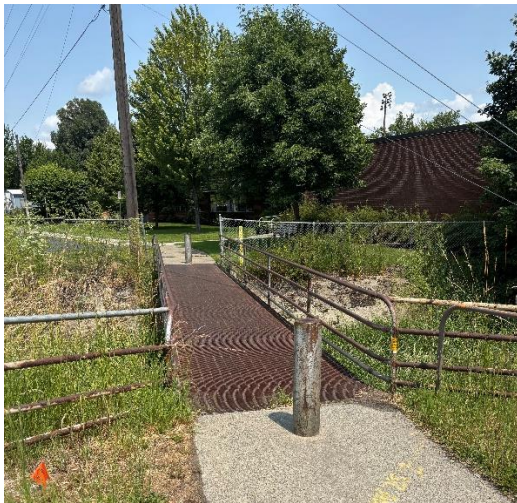
The existing Pedestrian Bridge at the southern extent of Home Street. The bridge deck is too narrow, sits too low within the flood plain, and the handrails/guardrails are not code compliant and are unsafe.
