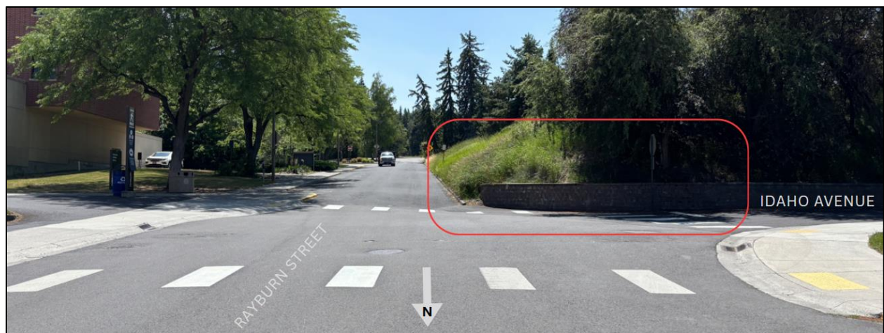
Existing conditions show the hillside needs to be cut and pushed back with a more substantial retaining wall in order to allow pedestrians to be seen by oncoming traffic
