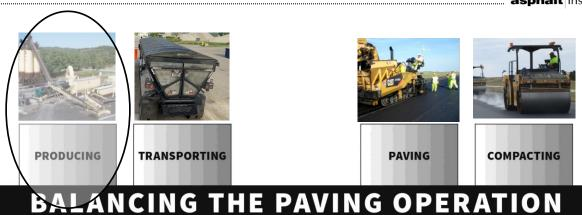
The synchronized balance of the four phases of asphalt paving to provide continuous paving operations.
