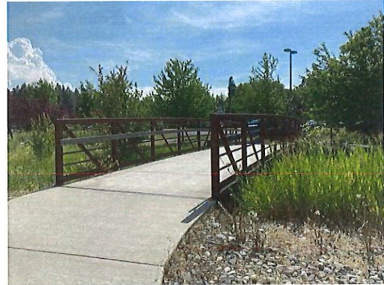
Existing Prefabricated Pedestrian Bridges spanning Paradise Creek.
