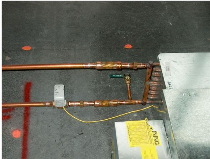
Typical fan box coil piping connection 02
