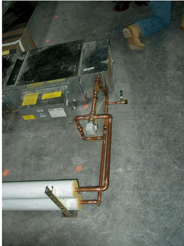
Typical fan box coil piping connection 01
