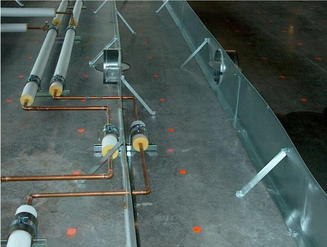
Typical fan under floor piping and supply air chase ways
