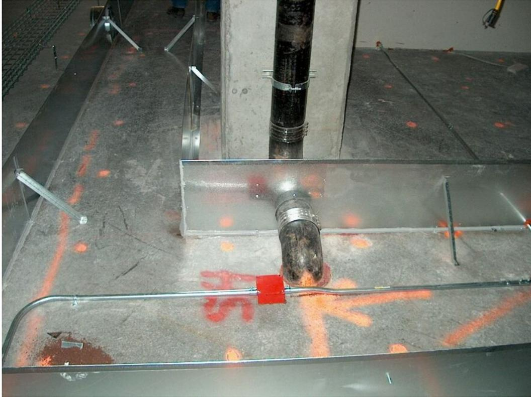
Typical RWL through underfloor air plenum divider
