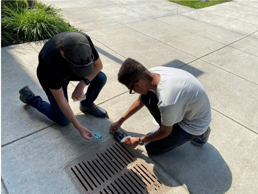
Figure 3: Stormwater drain labels read "DUMP NO WASTE; DRAINS TO STREAM"
