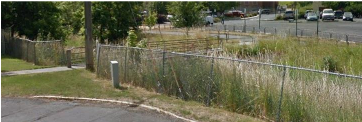
The existing Pedestrian Bridge at the southern extent of Home Street. The bridge deck is too narrow, sits too low within the flood plain, and handrails/guardrails are not compliant and unsafe.
