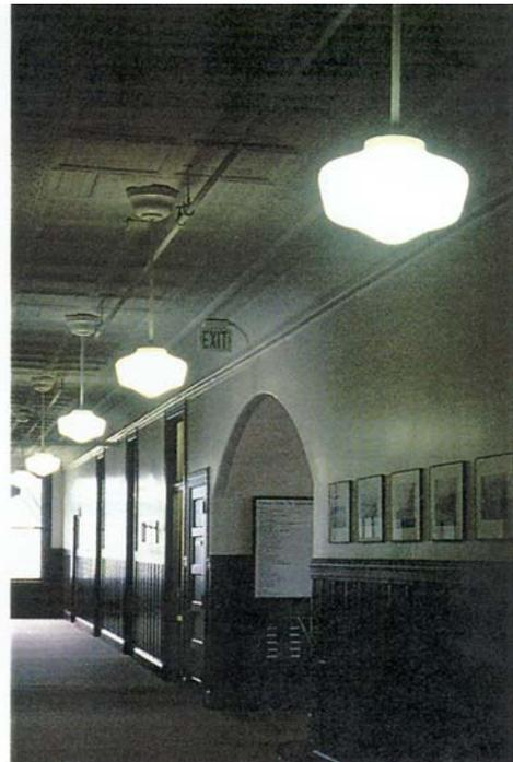
*A simple, historic styled light fixture, such as the contemporary manufactured one shown above, is one approach to lighting design for the building. Lamps can be energy-conserving types.*
